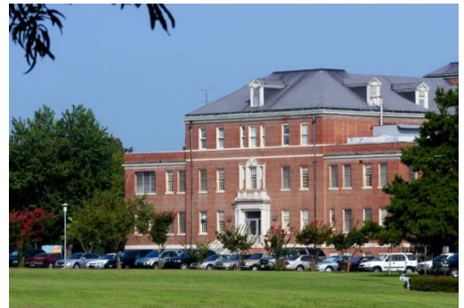
The SC MIRECC fellowship is located in building 58 at CAVHS.
